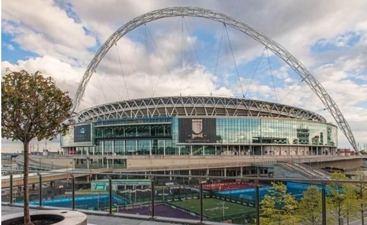
The view from our level 3 terrace
